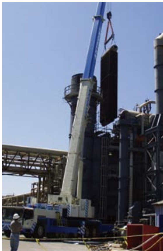
1. The newest HRSGs incorporate design improvements—such as elimination of tube bends between headers and superheaters made of P91/T91 material—to boost HRSG durability and reliability. But existing plants also can achieve improvements through O&M modifications
